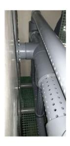
PCM tank stores the waste energy from the heat pumps while the heat pump is utilised for the heating services. Building is provided with approx. **1,500 kWh(426 ton-h)**
